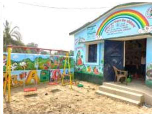
AWC - After Renovation
