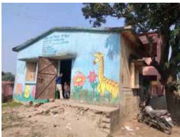
AWC - Before Renovation
