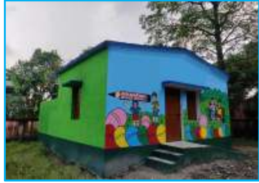
AWC - After Renovation
