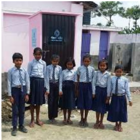
Finished Toilet at the Primary School
