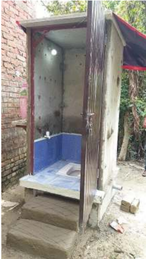
Finished Toilet at HH3
