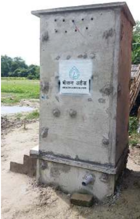
Finished Toilet at HH1
