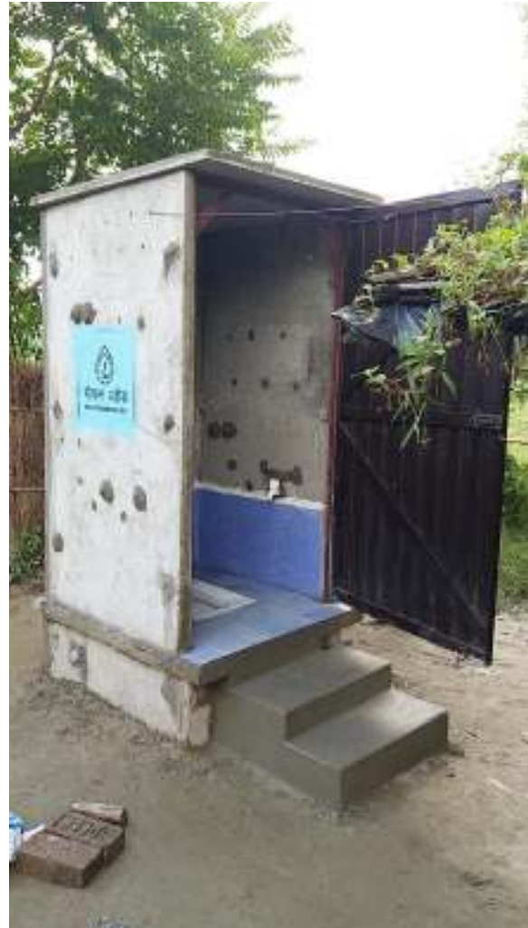
Finished Toilet at HH2
