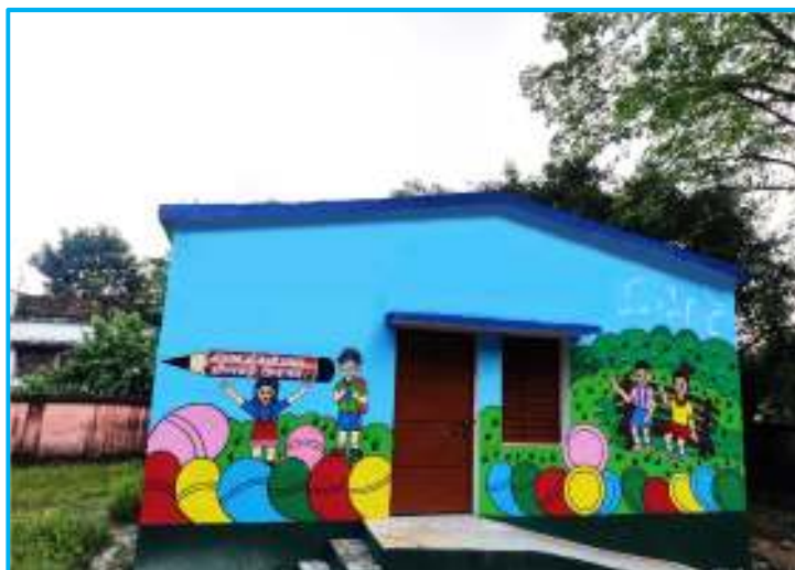
Renovated ICDS Anganwadi Centre
