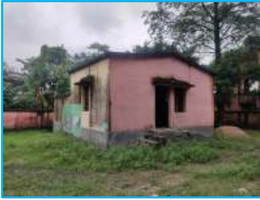
AWC - Before Renovation
